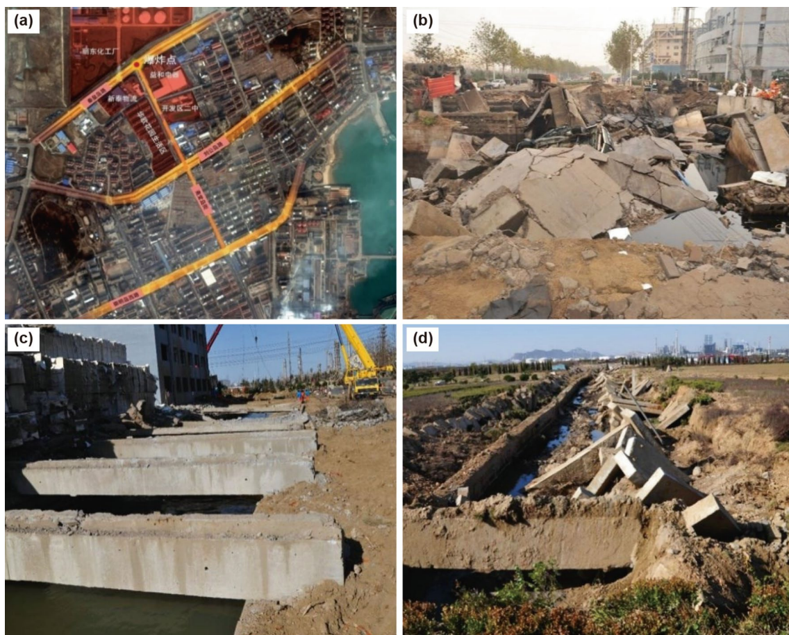
Fig. 2 Scene photographs of the explosion site a bird view of the location of the explosion point, b scene of the oil spill point after explosion, c scene of the nearby street, d scene of the drainage of the adjacent plant
